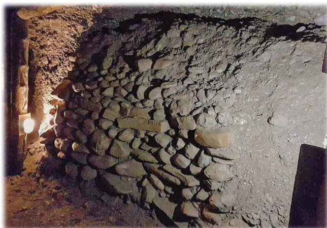
Figure 6. Dry-stone wall constructed within a tunnel passage, composed of river pebbles and used to block or stabilize a sealed section of the underground network.
